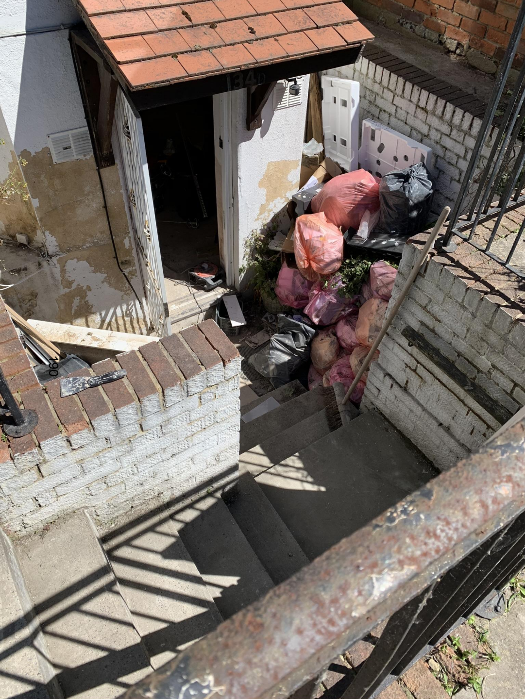
Example of comparable arrangement at attached neighbour No.134
